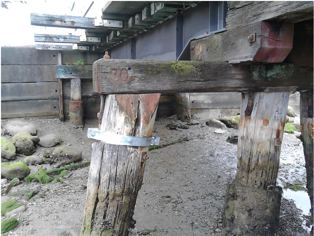
The first new clamp has been fitted.
